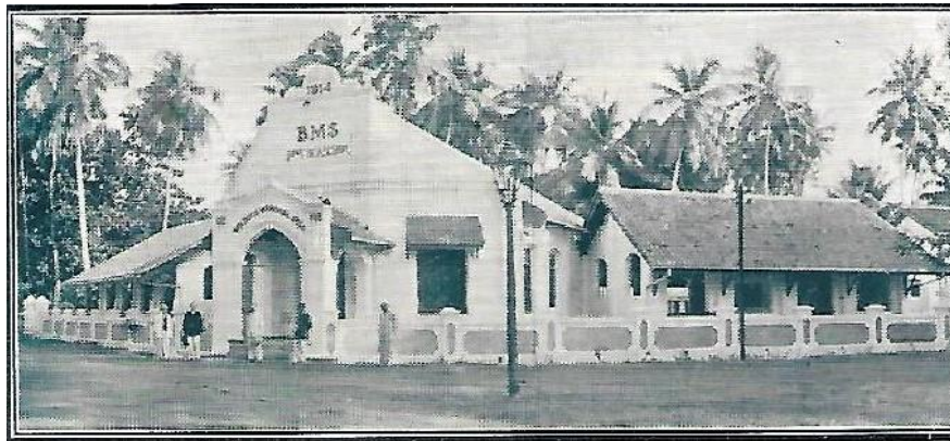
“CENTENARY HIGH SCHOOL & WALDOCK MEMORIAL HALL.”
